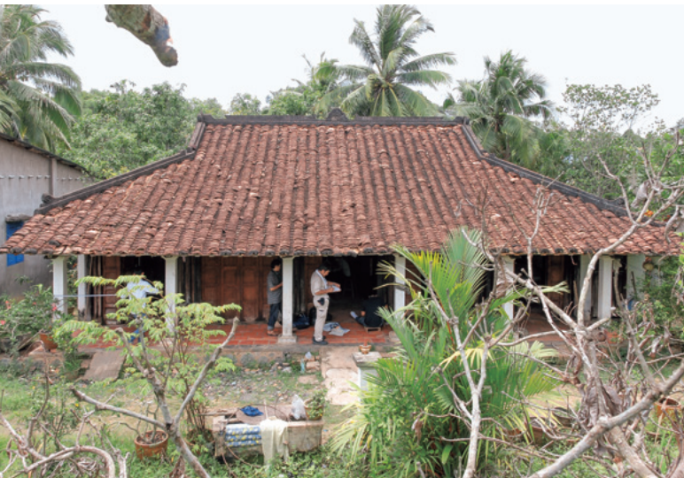
建造物研究室：ベトナム・フーホイ村の集落調査 Architectural History Section: Community investigation at Phu Hoi Village, Viet Nam
