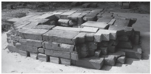
Fig. 74: Trial assembly of the upper foundation (viewed from the northwest)
